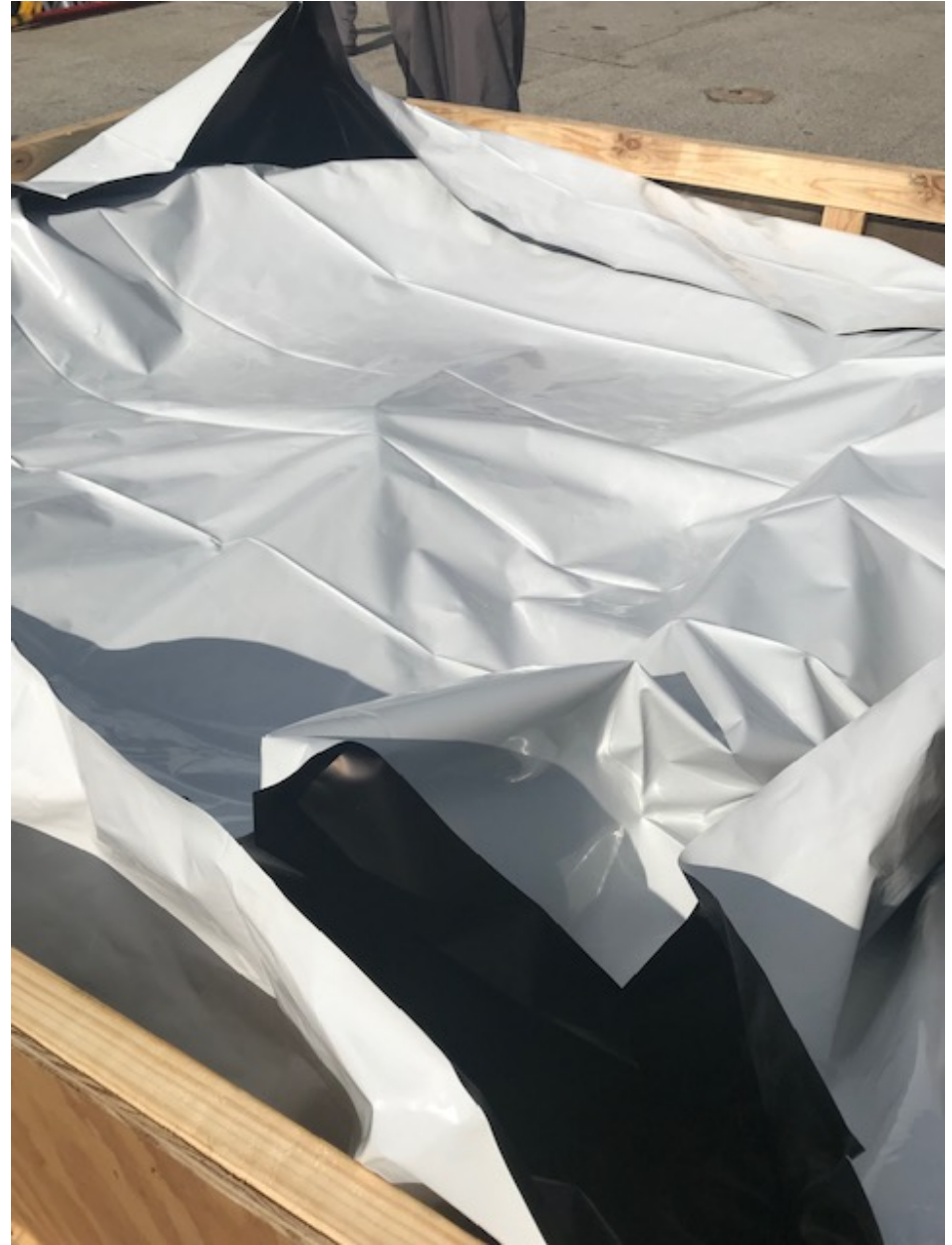
Once the unit is desiccated, apply the Intercept top-sheet over the bag, as shown in the picture on the right.
